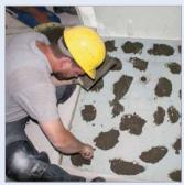
Using mortar dots uneven surfaces can be levelled off quickly and without great effort and the shower element can be installed precisely horizontally.
