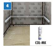
Adhere the support strips in the correct position to the surrounding walls.
